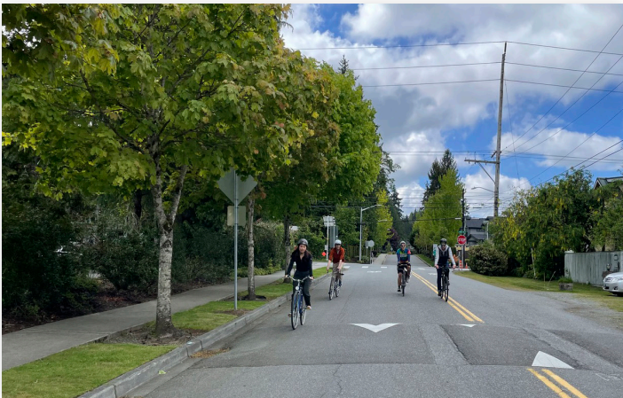
Road safety improvements using speed humps
